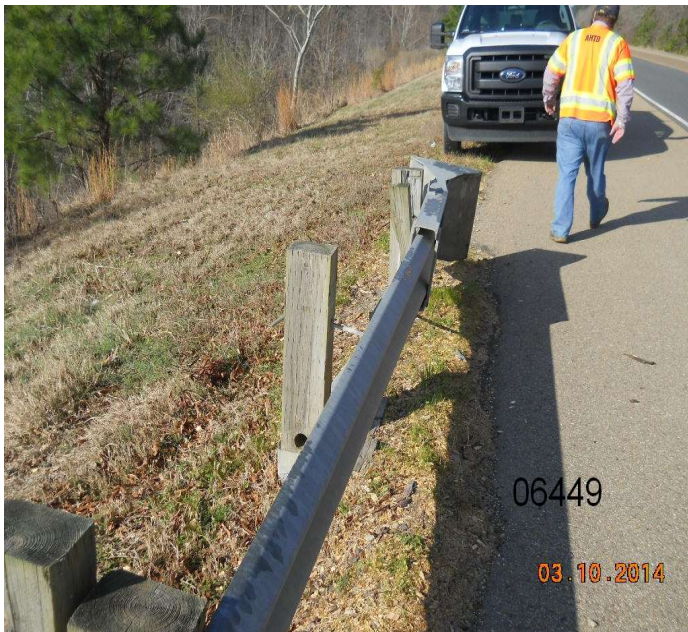
PHOTO 1 Description Abutment 1 Rt. side terminal end post and spacer block broke.
